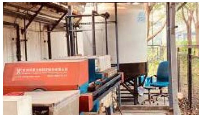
The Suzhou, China site initiated a wastewater optimization project that reduces sludge disposal weight by 50% each month, reducing the annual disposal weight by 12 metric tons. The project consisted of adding a buffer tank for sanitary sewage. After sedimentation, the concentrated sludge is pumped into a pressure filter for further pressure filtration, removing more water.
